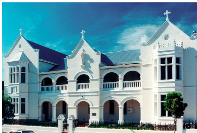
St Brigid's Convent, John Street, Northbridge (John Taylor, 2000)
